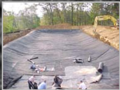
Liner Installation
