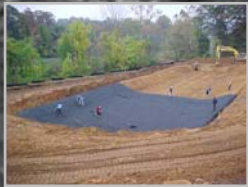
Geotextile Installation
